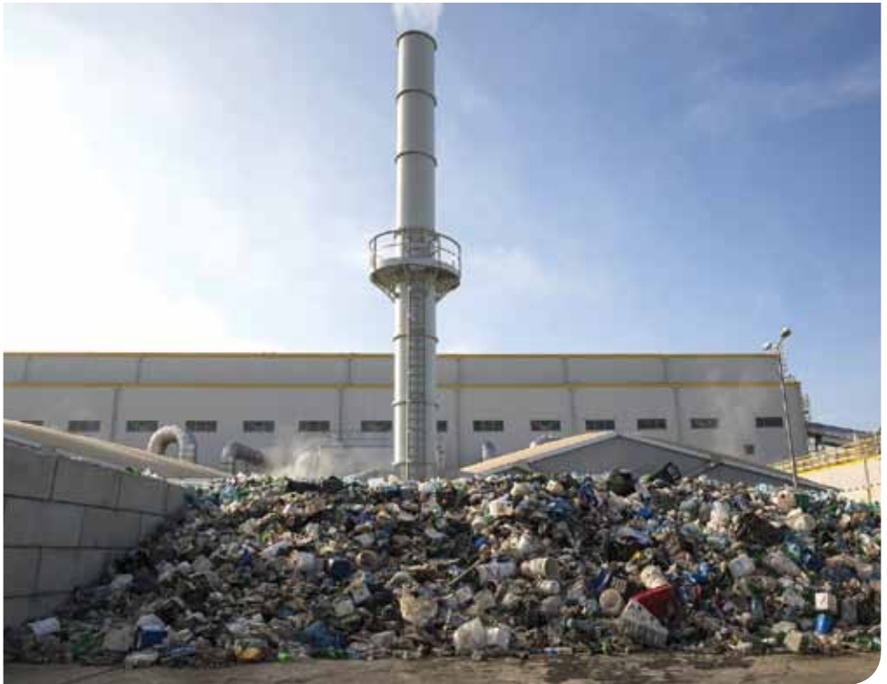
Energy-from-waste facility Image: Belish/Bigstock
